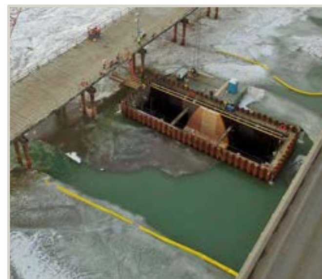
Figure 48, Example of a Cofferdam
