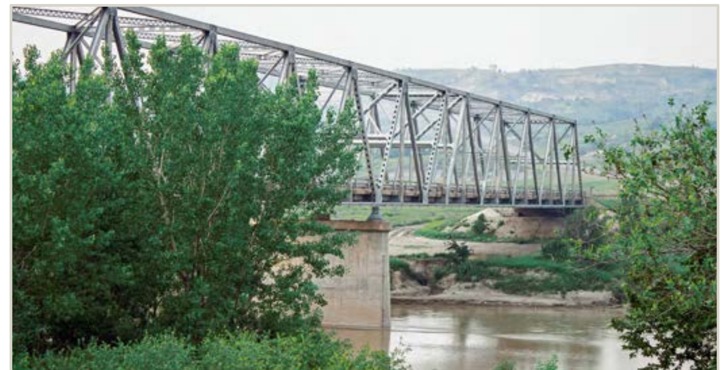
Long X Bridge (32MZ1807)
