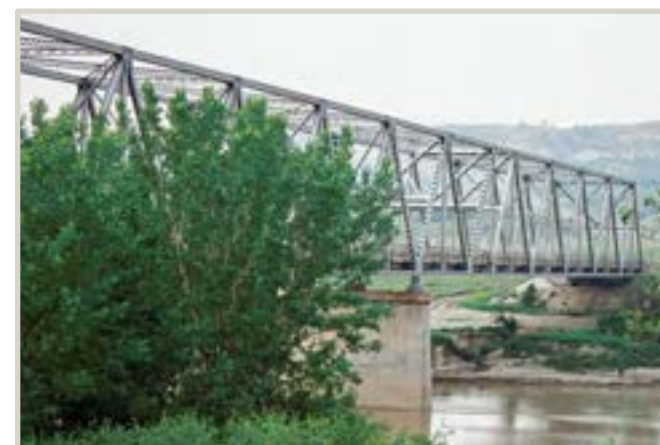
Long X Bridge (32MZ1807)
