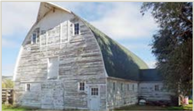
Architectural Features, Gothic-Arched Barn (32MZ3056)
