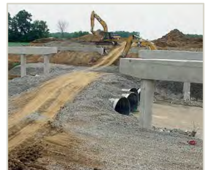
Figure 49, Example of a Causeway
