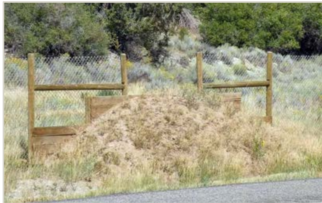
Figure 74, Jump-out Example (View from Highway)
