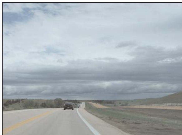
Figure 4 -- US Highway 79 Under Construction in South Dakota
